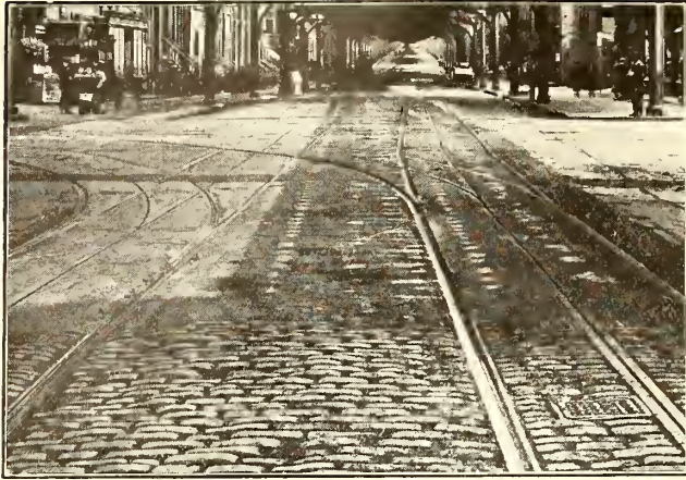
WEST BROADWAY AND CANAL STREET—CONTRAST FILLER AND KEY BLOCK CONSTRUCTION WITH GRANITE IN FOREGROUND
